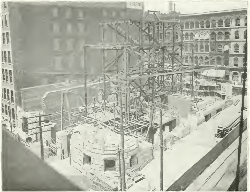
Early Stage of Construction, 1887, Showing Great Derricks.
